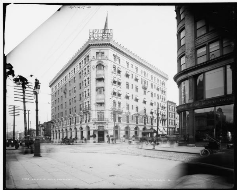
Bethune's opportunity to create a nationally significant building came in the early 1900s with a commission for the Lafayette Hotel. Located in downtown Buffalo, the seven-story, 225-room Renaissance Revival hotel featured hot and cold water in all bathrooms and telephones in all rooms. It was praised as "one of the most perfectly appointed and magnificent hotels in the country" when it opened in 1904." ( "Buffalo Hotel Opened," The New York Times , June 2, 1904)
