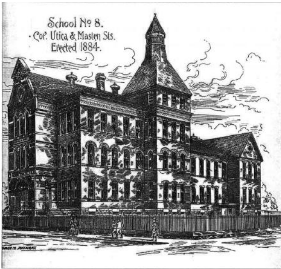
Bethune & Bethune Architects, Public School No 8, Buffalo, N.Y. Perspective sketch, 1884, published in Superintendent's Annual Report.
